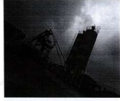
22&23. Photo of RMC plant
